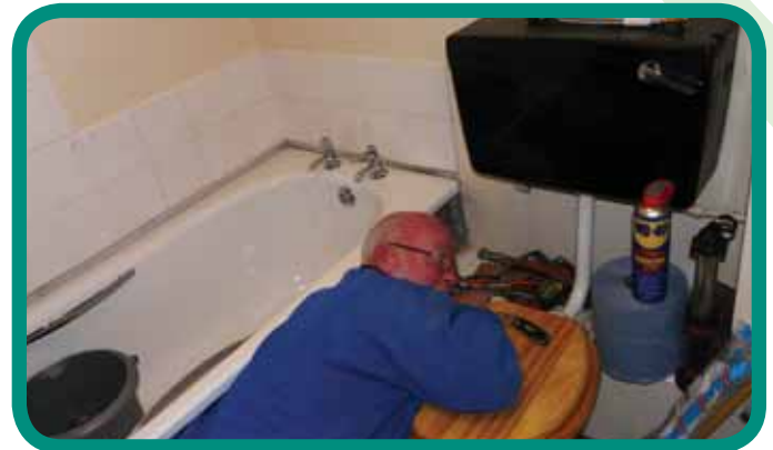
Eden Works carrying out repairs
